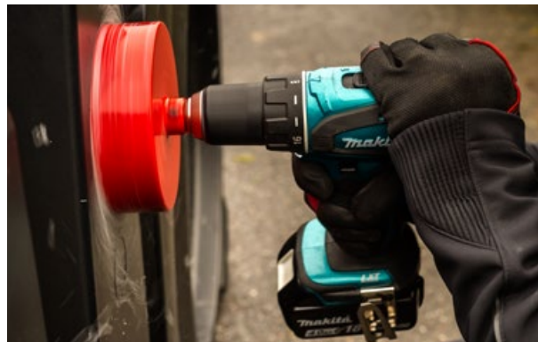
Make a hole at the bottom of the tank with the circle hole cutter to connect the retention throttle
