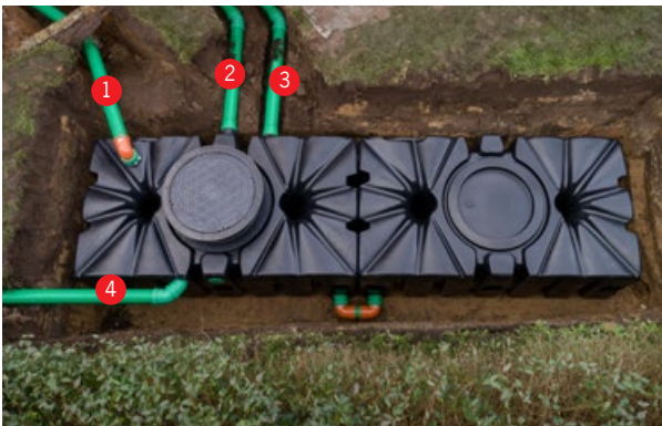
Example design of a 4,000 l rainwater tank used for retention and rainwater storage
