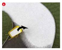
Fill in the GravelGuard tiles with 3-16mm gravel and compact. Once compacted add a further 15-20mm layer of gravel, finally rake the gravel to distribute evenly.
