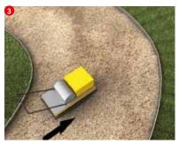
Compact the sub-base using a plate compactor. Fill the excavated area with free draining gravel or crushed stone to 110mm below the finished level. Tamp down with a roller or plate compactor.
