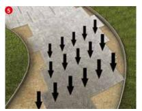
Install the ACO GravelGuard tiles along the length of the area. Install the tiles ensuring that the geo-membrane overlaps each other. For best performance the tiles should be laid in a staggered pattern rather than a grid pattern.
