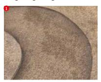
Depending on the soil conditions and intended use of the area to be stabilised, dig out the existing base. Typically, for driveways, 260-360mm. Note:
