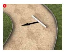
Level the area with a layer of fine sand to 60mm depth. Use a rail or wooden batten and compact.
